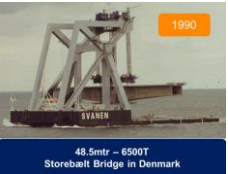
48.5mtr - 6500T Storebalt Bridge in Denmark
