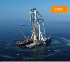
Modifications Extend gantry by +/- 25 mtrs. Upgrade spreader beams to 3000T WLL & 2000T WLL
