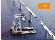
Modified 74.5 mtr - 8700T Pontons widened Construction of Confederation bridge Canada
