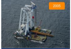
Modified for installation of monopiles and transition pieces:
